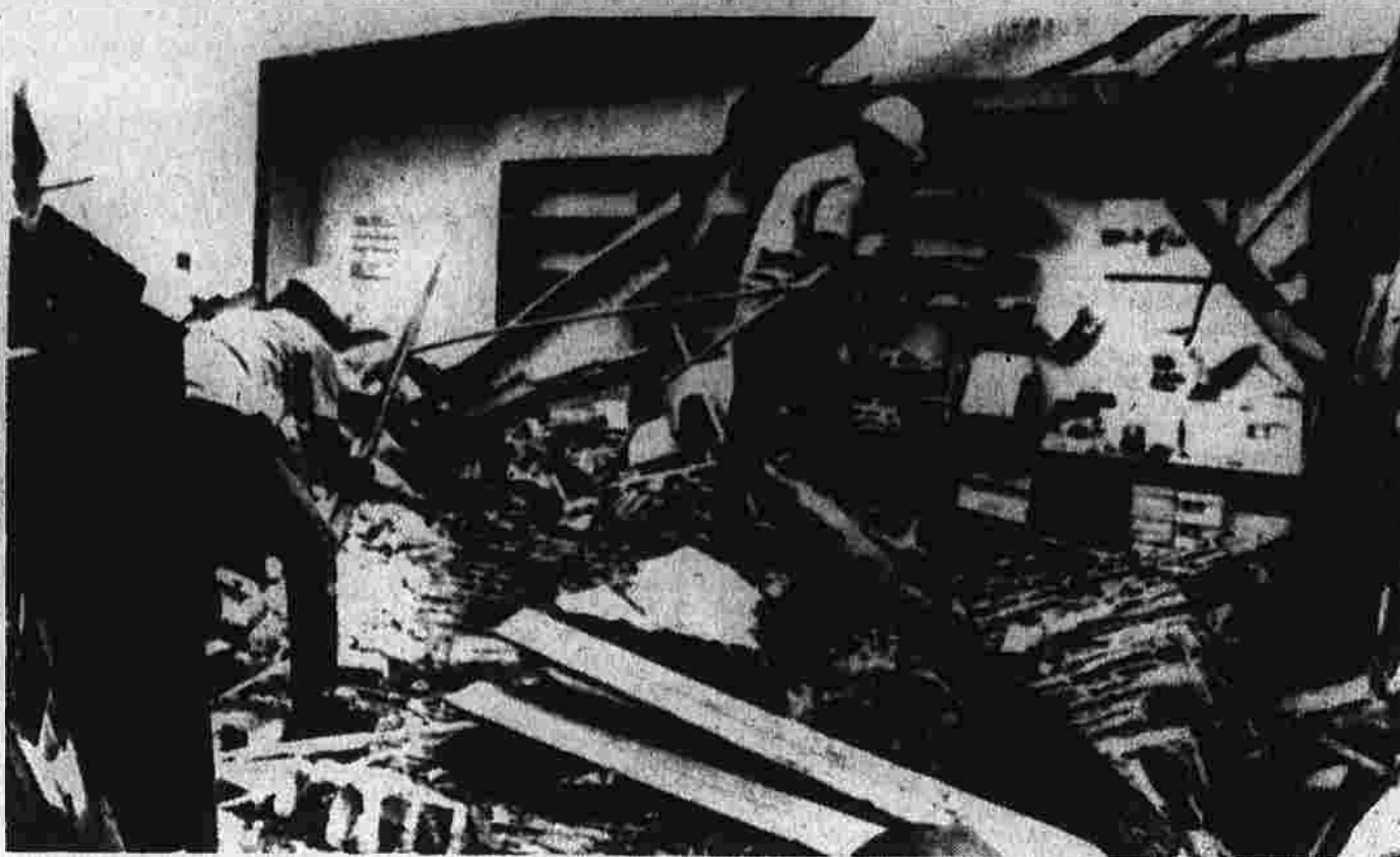
Workmen Clear Earthquake Debris
